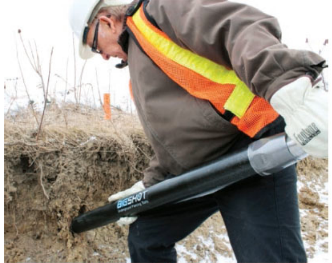
A contractor uses a Big Shot pneumatic piercing tool from Footage Tools on a job site. While piercing tools are some of the most durable pieces of equipment in the trenchless industry, contractors should still perform regular maintenance on them.
