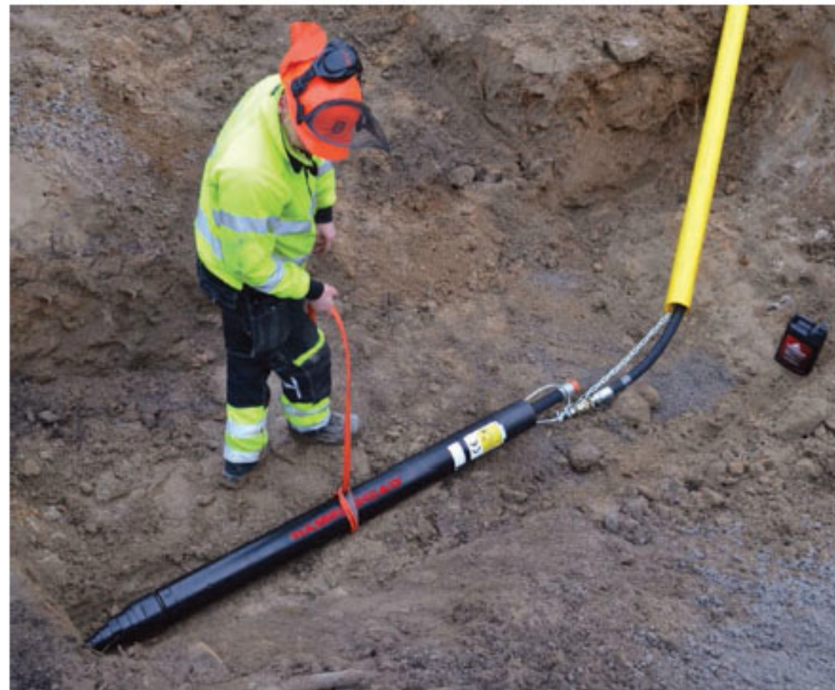
A contractor sets up a HammerHead Trenchless pneumatic piercing tool on a job. Manufacturers say the best things to remember when it comes to the tools are to clean it, lubricate it and store it correctly.
